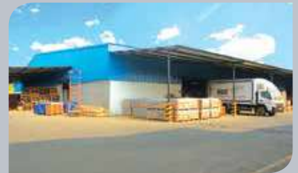
Covered Carting & Stuffing Area
